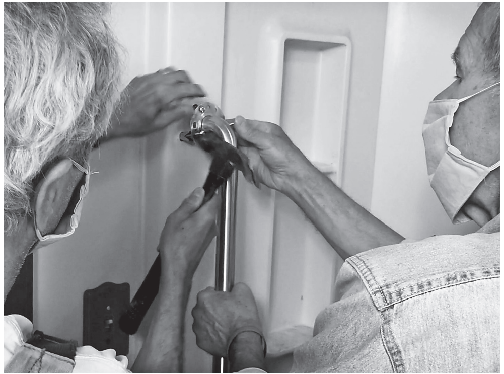
Two NHCO volunteers install a grab bar in the shower at a senior's home during a home safety check.
